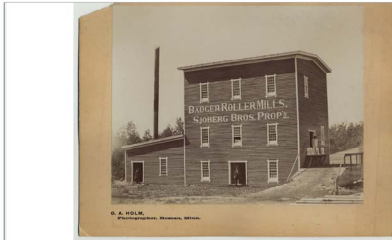
Title Badger Roller Mill, Badger, Minnesota Creator Holm, Ole Alex, 1869-1950 Contributor Holm Studio (Roseau, Minnesota) Description Exterior view of the Badger Roller Mills, the Mill was owned by Sjoberg Brothers.
